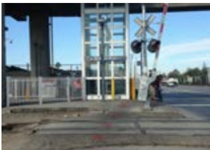
Slauson Station pedestrian access involves an at-grade railroad crossing to enter the elevated Blue Line platform.
