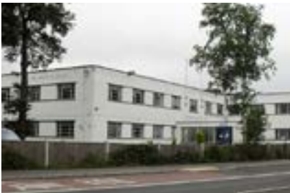
Example of an industrial operation fully enclosed in a building.
