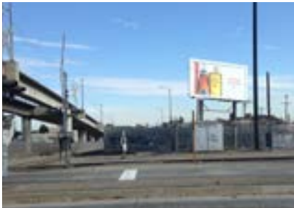
Poor pedestrian amenities at Slauson Station.
