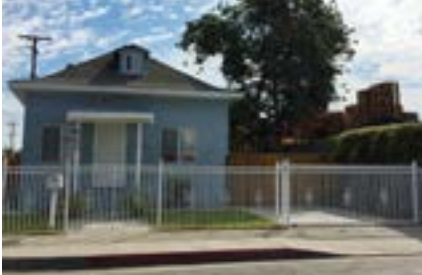
Industrial use adjacent to residential use.
