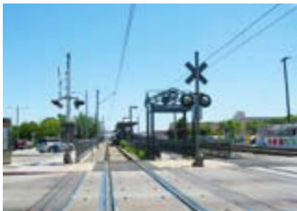
Florence Station is the only Blue Line station located at street-level and has a great opportunity to safely connect to the surrounding areas.
