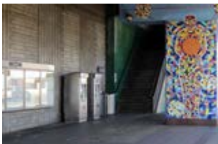
Firestone Metro Station.
